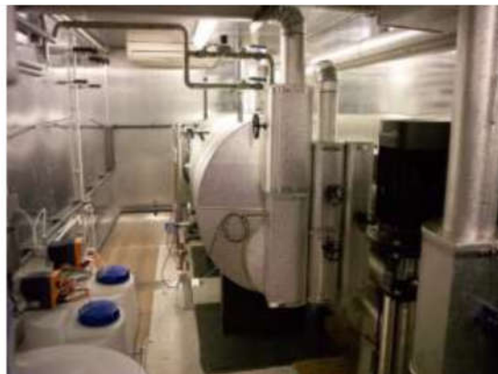
Feed Water Tank in Container
